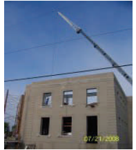
Adding the roof.
